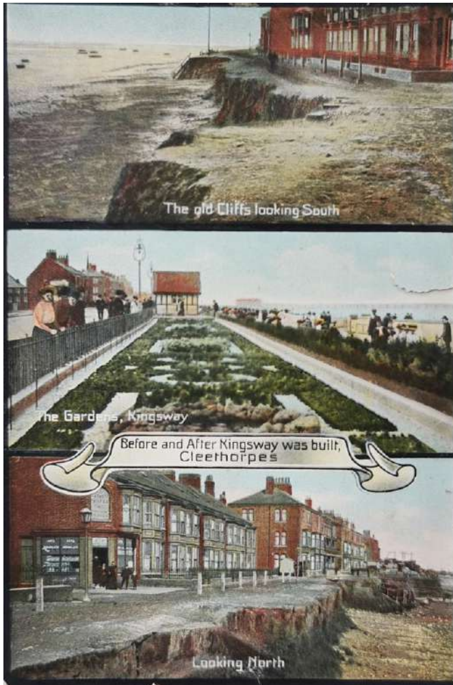
Figure 120: Before and After Kingsway was built at Cleethorpes, from an early twentieth-century postcard, showing the low cliff being eroded towards the houses here.
