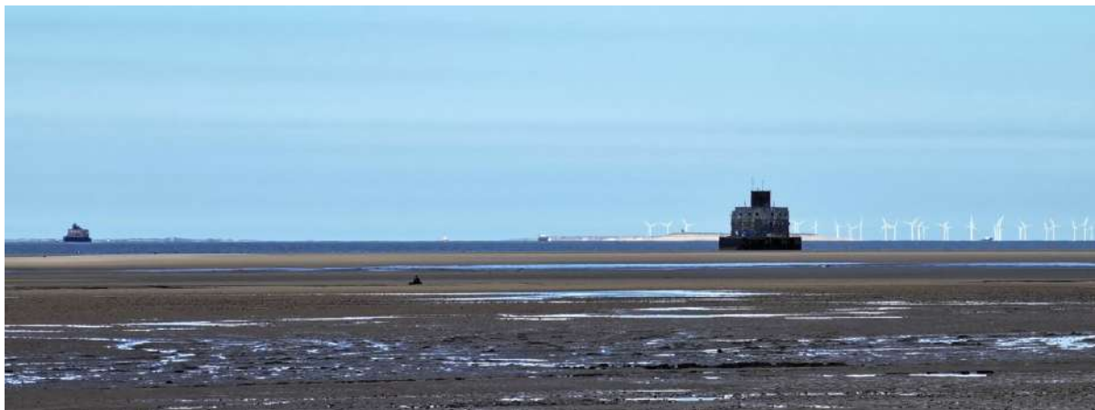
Figure 135: The two great Humber Mouth forts, Bull Sand Fort (left) and Haile Sand Fort (right), with Spurn Point in the background; begun in 1915, they were completed too late to be of much use in the First World War but were used in World War Two.
