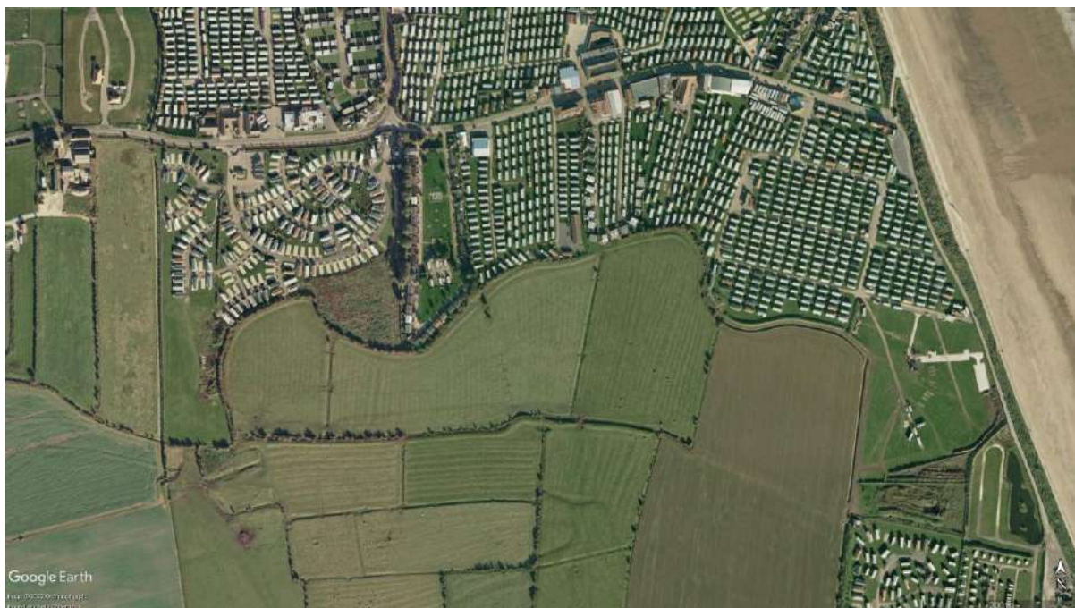
Figure 108: The mouth of the Schalflet on the coast between Chapel St Leonards and Ingoldmells. The line of the creek here is nicely preserved by field boundaries and a bank to the south and Trunch Lane to the north; the creek itself is covered by late medieval ridge and furrow in the south and a caravan park in the north (Source: Google Earth image from 2006, Maps data © 2022 Google, Image © 2022 Getmapping plc Image Landsat/Copernicus).
