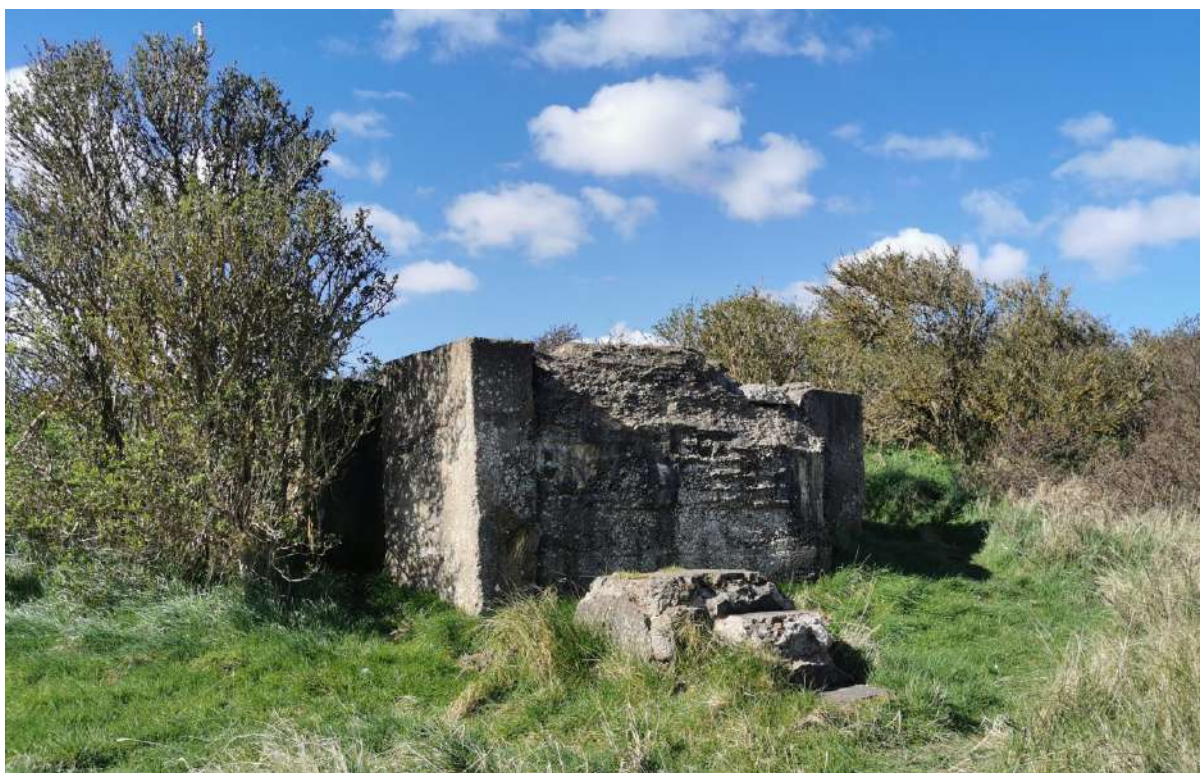
Figure 136: A First World War pillbox at Sea Lane, Saltfleet, probably built in 1917. This forms part of an organised system of coastal defence, with pillboxes placed in this area at regular intervals. It had a convex curved roof at least 1m thick and sandbag shuttering as part of an attempt to make it resistant to naval bombardment. It was probably manned by soldiers of the 7th/8th Battalions of the Sherwood Foresters in World War One; at the outbreak of the Second World War, the pillbox was reoccupied and integrated into the new anti-invasion defence, and it is now a Grade II listed building, no. 1445089.
