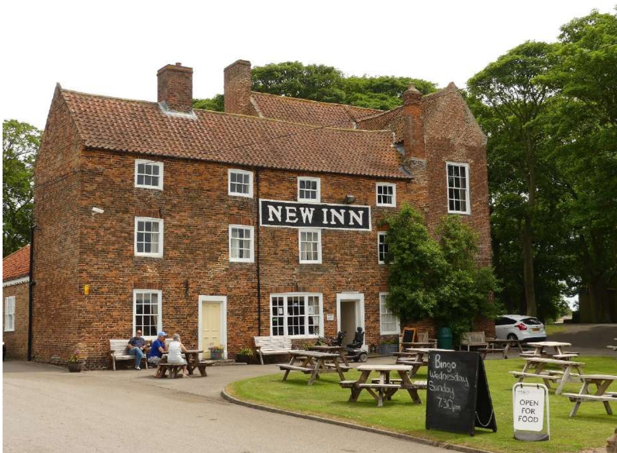
Figure 52: The New Inn at Saltfleet. This is a substantial seventeenth-century T-shaped building, the ‘Old Inn’, with a new additional north wing built in the later eighteenth century, leading to its renaming; it has been suggested that the original ‘Old Inn’ had its origins in the late sixteenth century.
